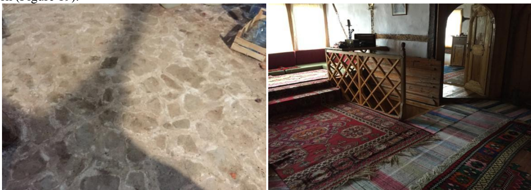
Figure 19: Floor covering on the ground floor (“magaze”) are stone slabs (left) and floor covering in the first floor (chardaks and sofas)
