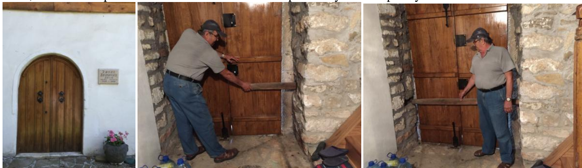
Figure 23: Entrance door to the house. Entrance door closing mechanism (wooden beam-mandal)
