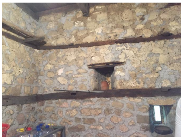
Figure 16: Construction and materialization of the ground floor wall Source: Autor (07.22.2016.)
