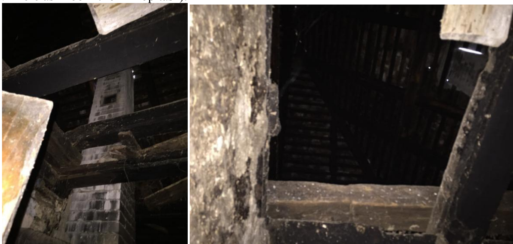
Figure 18: Roof construction Source: Autor (07.22.2016.)
