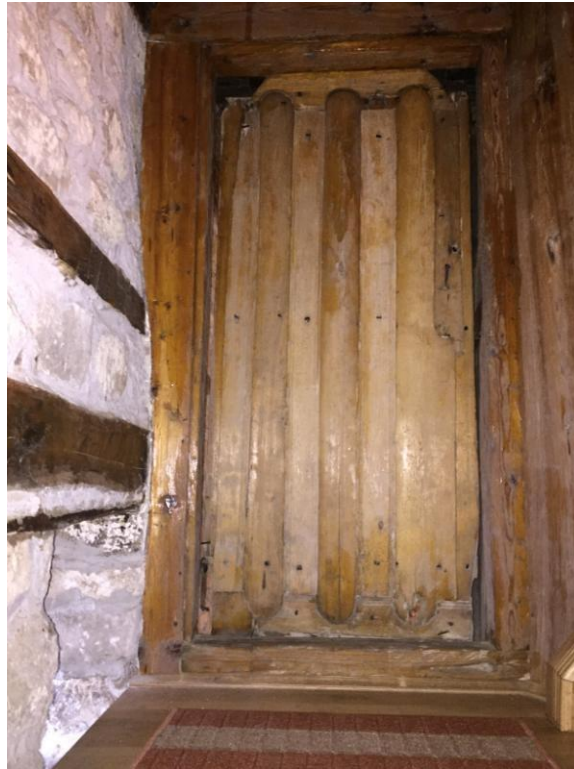
Figure 25: Original pantry door (accessed from the stairwell landing) Source: Autor (07.22.2016.)
