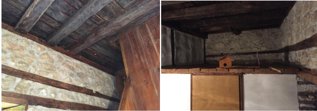
Figure 20: Preserved original mezzanine structure ground floor-first floor Source: Autor (07.22.2016.)
